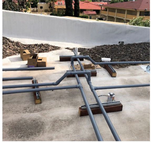
Leveraging the expertise of Integrity Plumbing's senior techs, test stacks of the two-story structure were created to validate the piping route that could bypass the ceilings.
