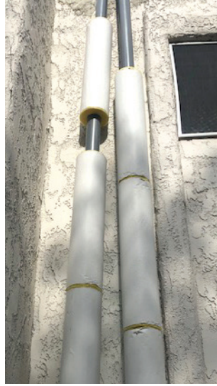
Leveraging the expertise of Integrity Plumbing's senior techs, test stacks of the two-story structure were created to validate the piping route that could bypass the ceilings.
