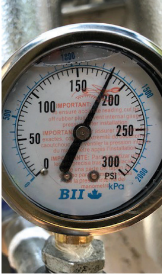
The solvent welded joints were pressure tested to 190 psi.
